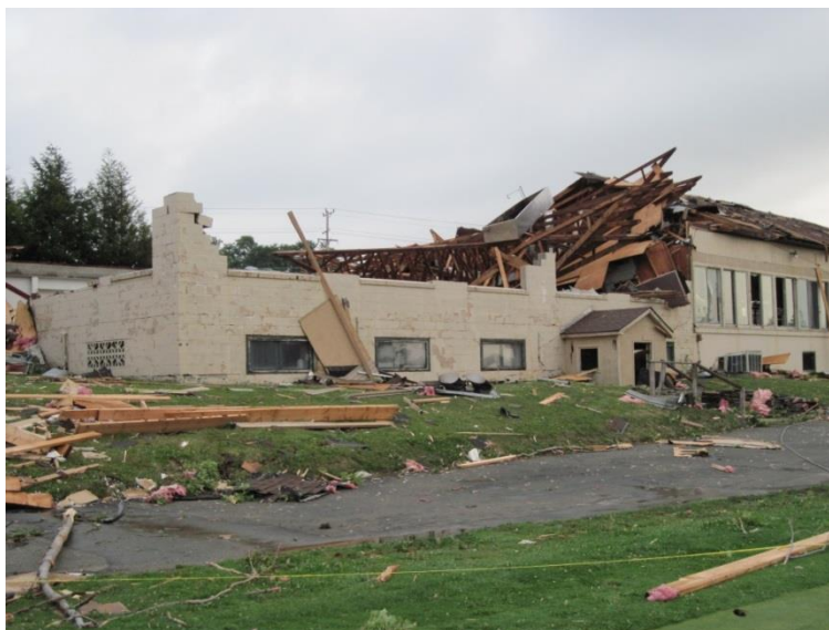
Tornado damage in Chautauqua County
