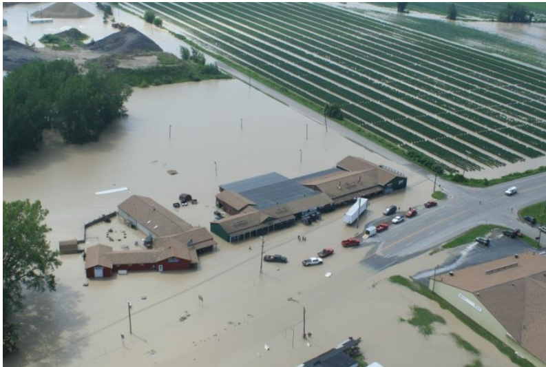
Flood damage in Chautauqua County
